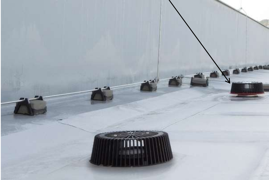
Dallmer 65 SuperDrain (note secondary system outlet in background)
