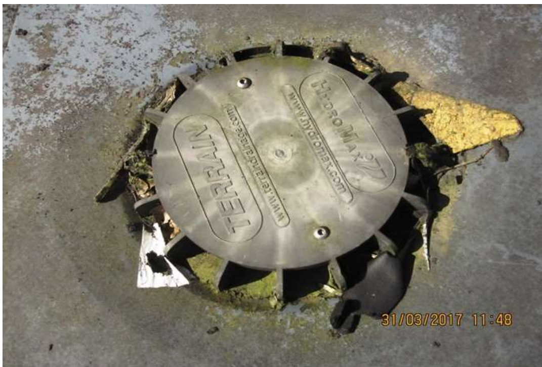
Polypipe Terrain/Hydromax (installed)
